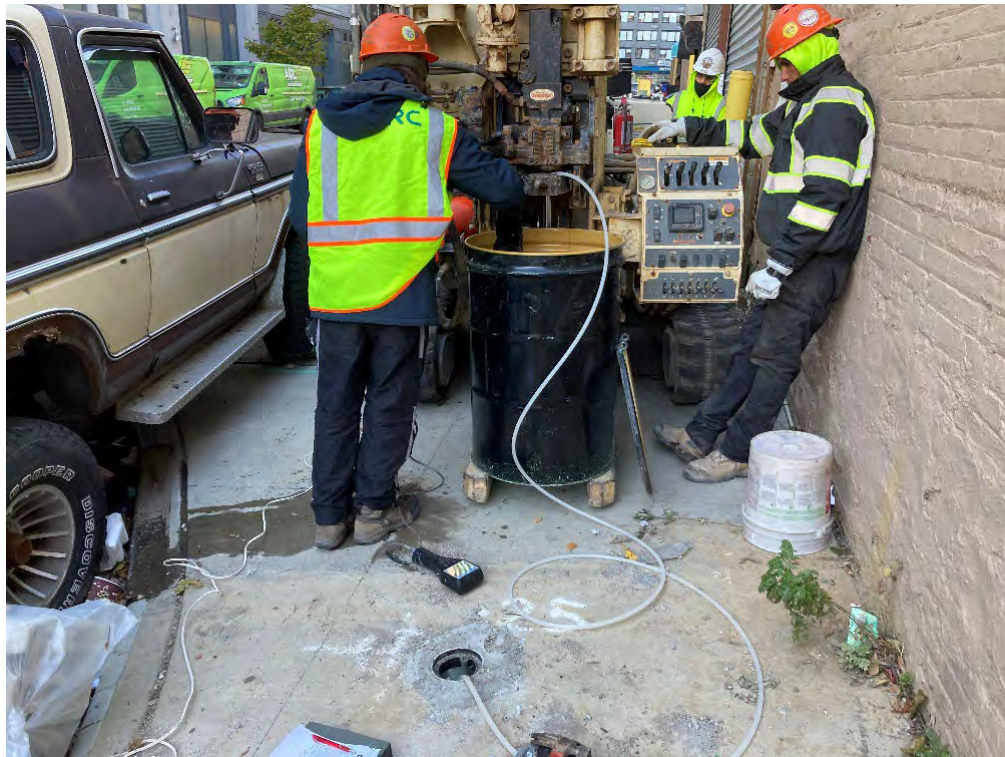
Photo 8: Development of monitoring well, TRC-MW-25, typical.
