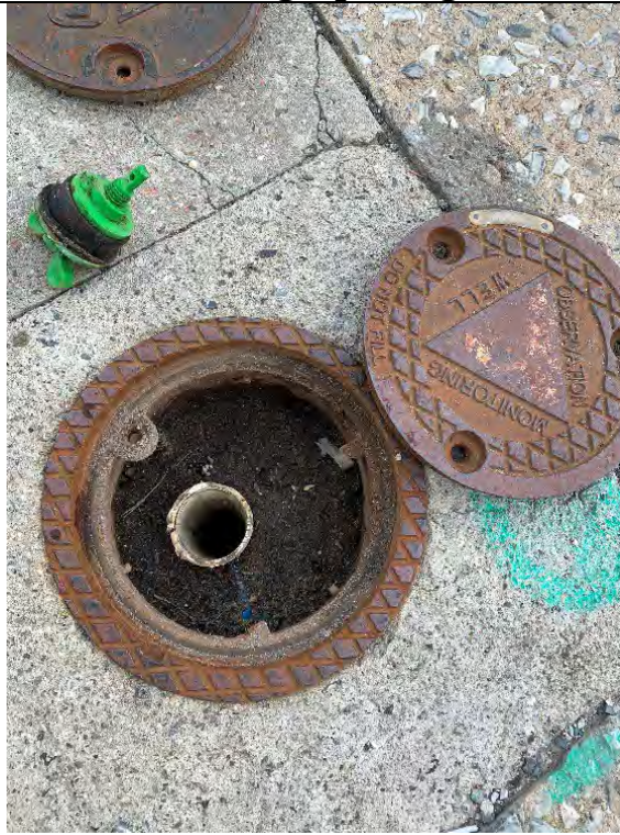
Photo 11: View of existing monitoring well, RMW-3, located in the northern portion of the Site.
