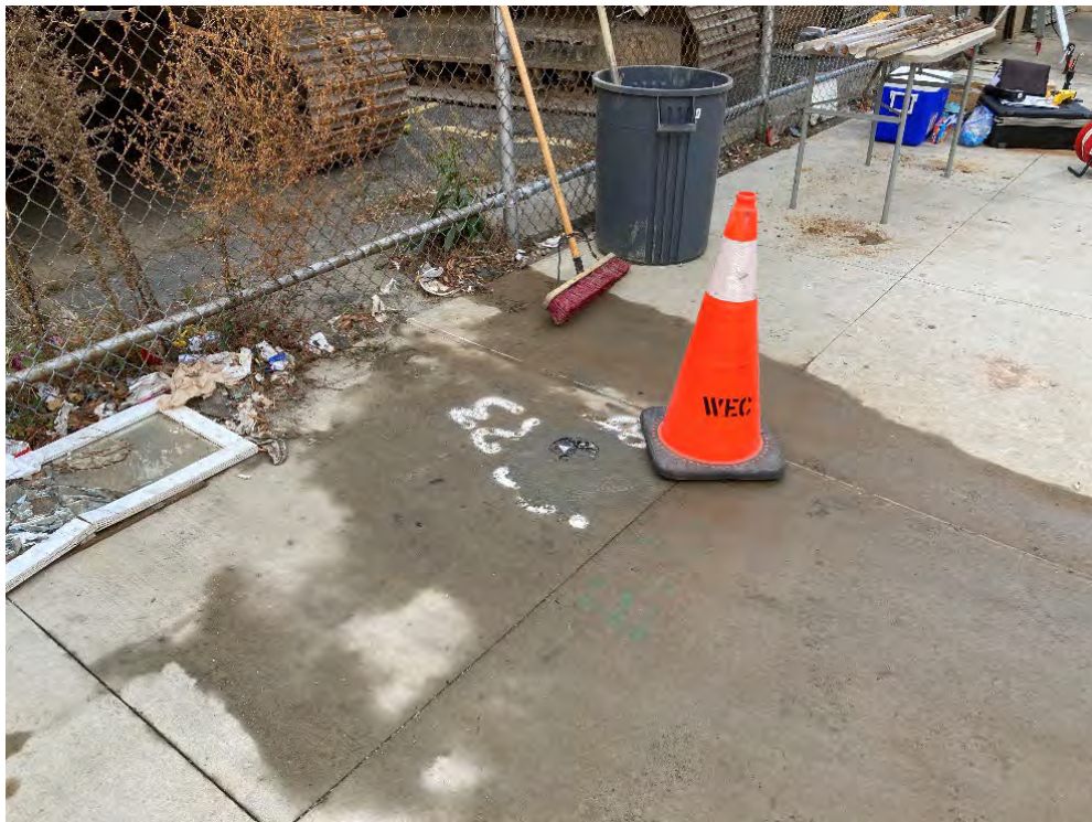
Photo 4: Flush-mount 2-inch diameter monitoring well installed at TRC-MW-23.
