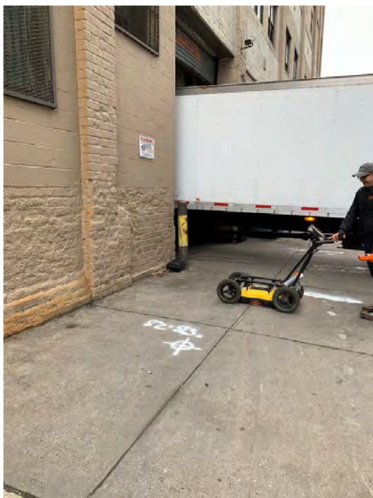
Photo 1: Geophysical survey at proposed soil boring location SB-28, typical.
