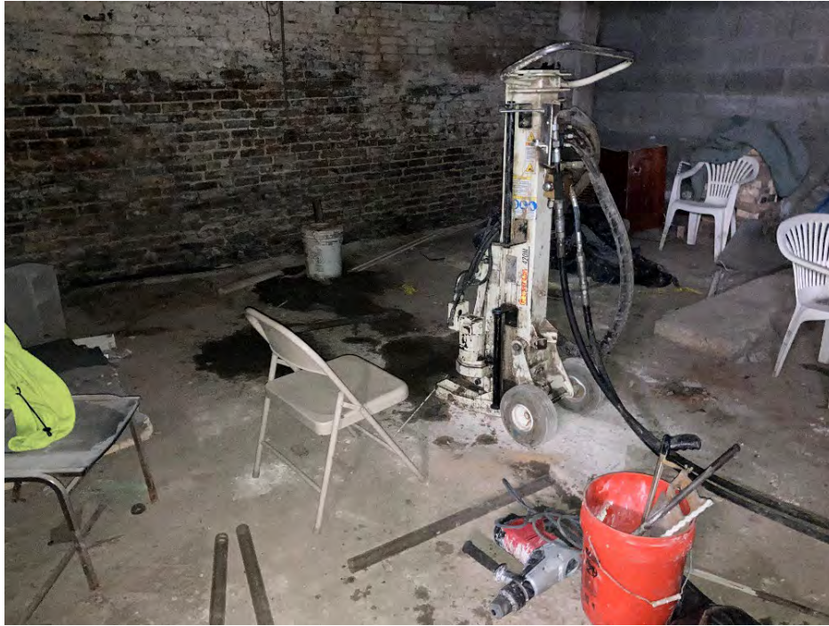
Photo 9: Advancement of soil boring, SB-02-N2, using Geoprobe 420M drill rig.
