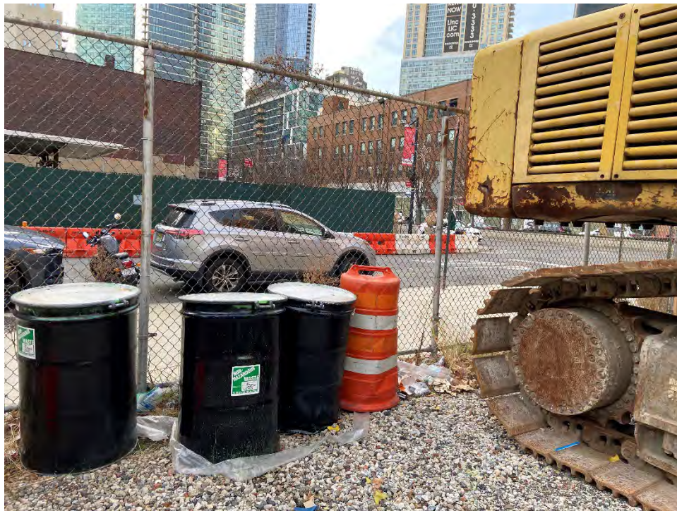
Photo 12: View of 55-gallon drums containing purged groundwater and soil cuttings, located in the northwestern portion of the Site to be removed.
