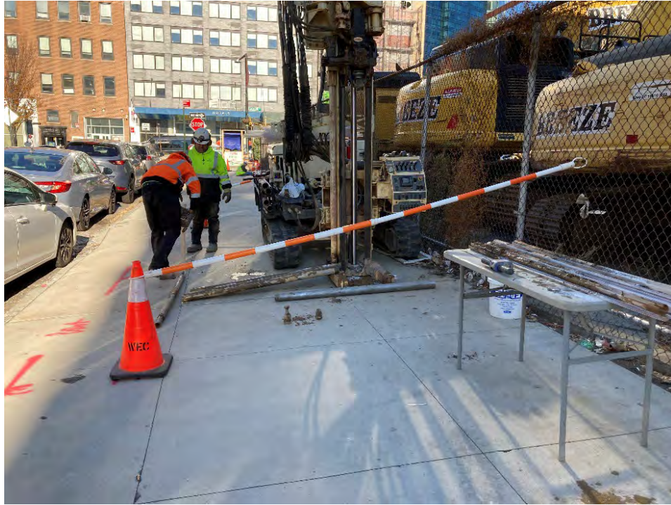
Photo 3: Advancement of soil boring, TRC-SB-23/ MW-23 along Queens Street sidewalk.
