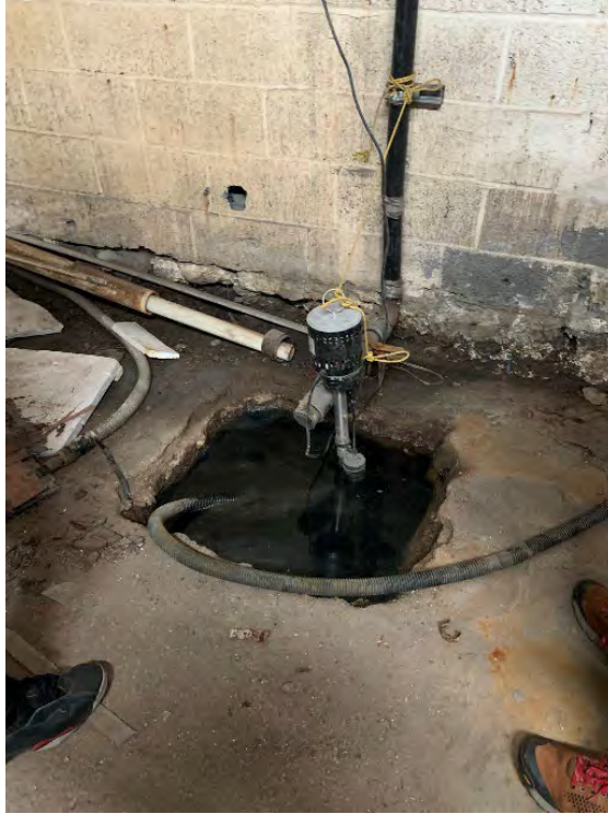
Photo 15: Building Sump 03, typical.
