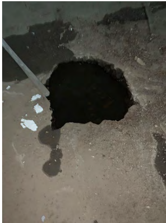
Photo 14: Slab Opening 02, typical.
