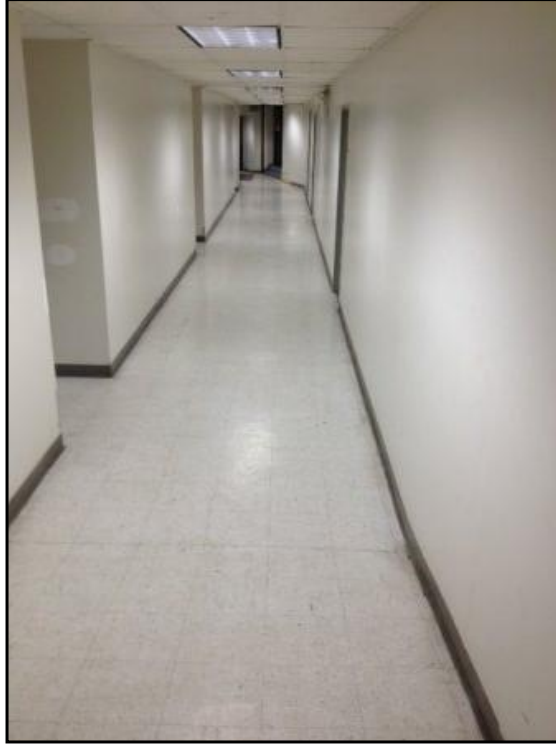
The second floor of the on-Site building consists of offices.
