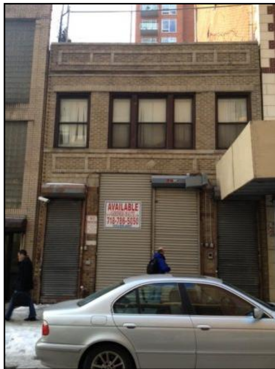
A north adjacent lot is occupied by a vacant 2-story building.
