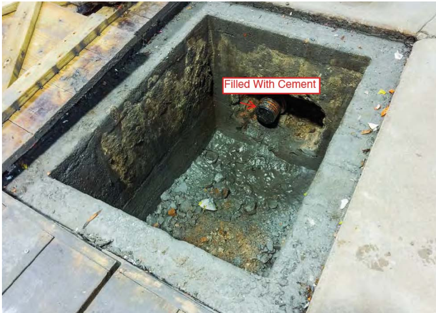
Figure (6) Below shows point source pipe with a sheen in the soil.
