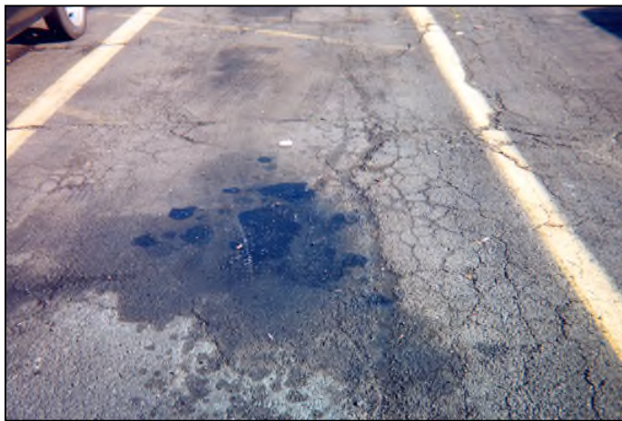
Photograph 7. Oil staining and cracks in asphalt pavement of Commercial Truck Parking lot.
