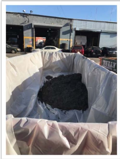
5. Placing Contaminated Soil into 20-yards Container
