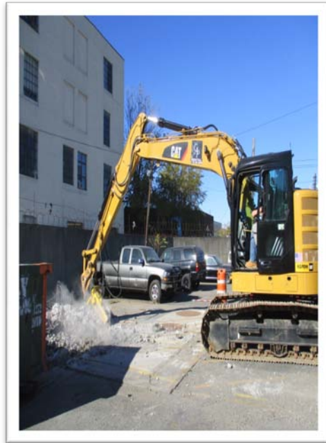
2. Breaking up the Concrete by Utilizing Excavator
