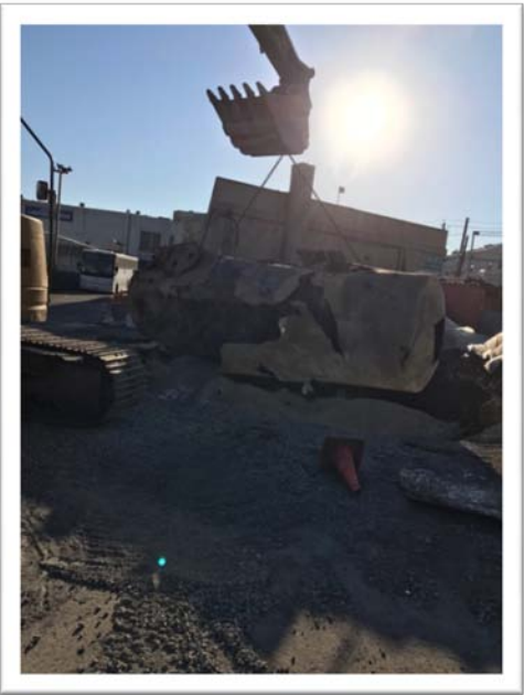
19. Lifting the Tank for Transportation
