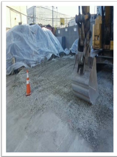
15. Backfilling the Excavation Area with RCA to the Ground Level
