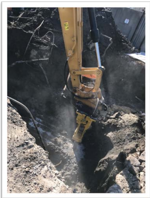
7. Breaking up the Concrete Around the USTs Location
