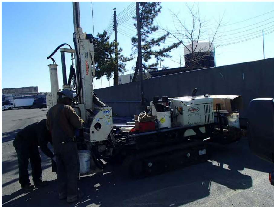
Photograph 4: View of a boring location along the northwest property perimeter.
