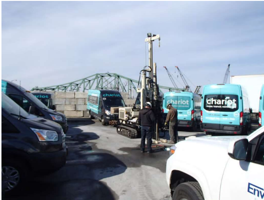
Photograph 5: View of boring location GP-8 at the northwestern corner of the property.
