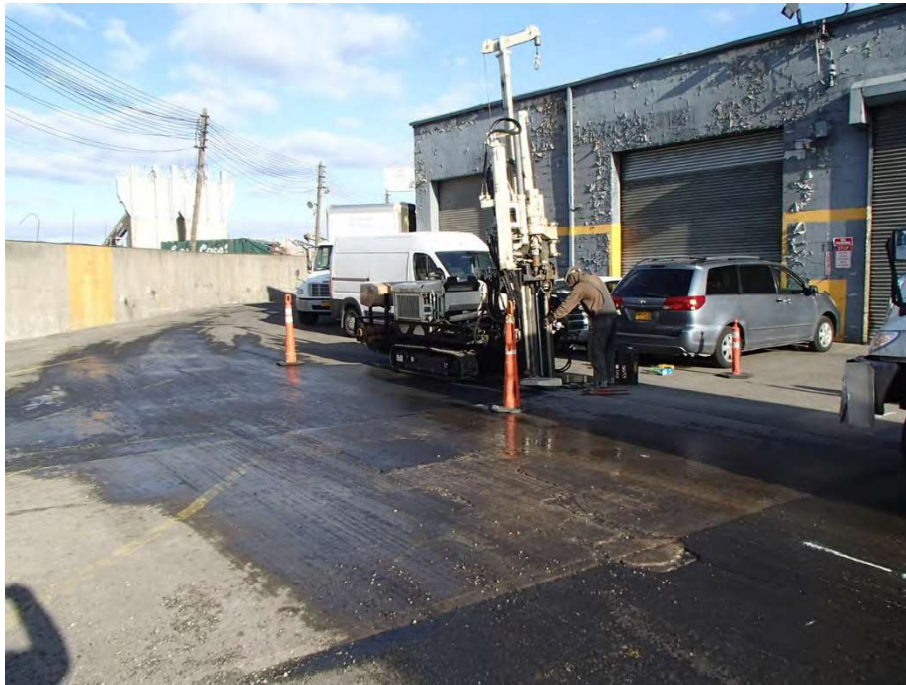
Photograph 1: View of the boring location GP-2 located to the north of the garage.
