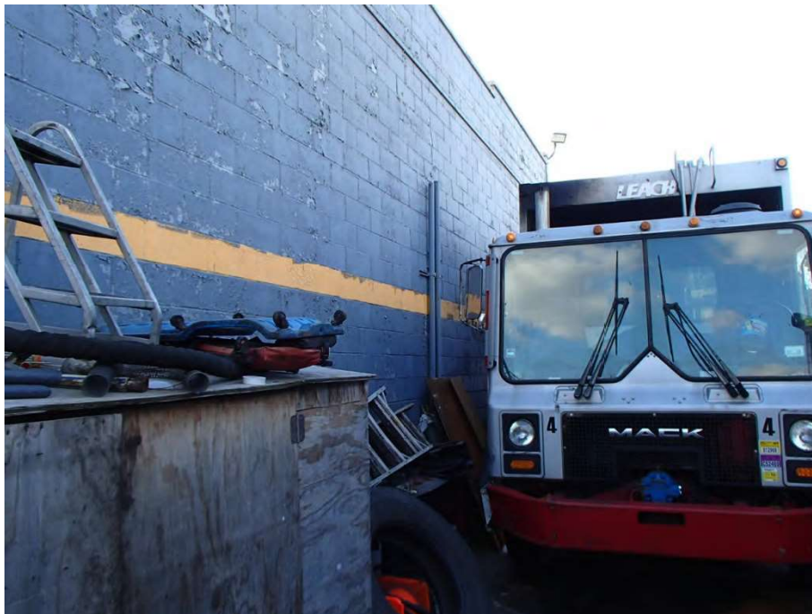
Photograph 2: View of the two (2) vent pipes associated with the oil-water separator located to the west of the garage.
