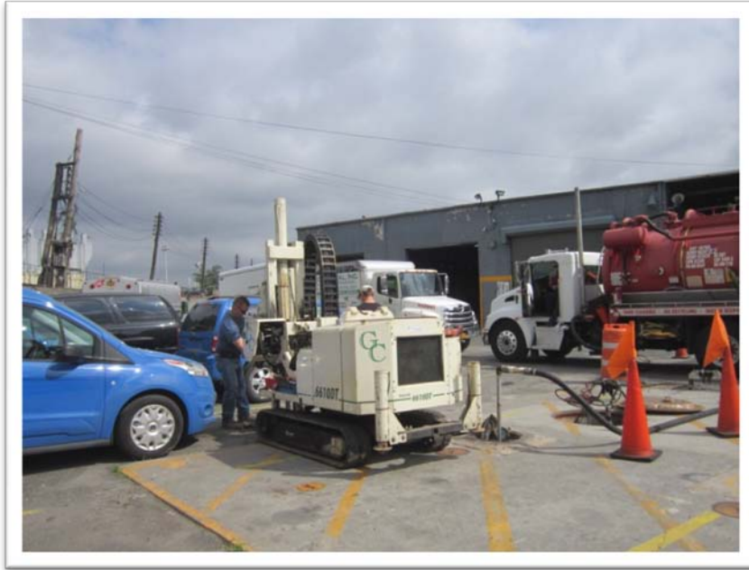
7. Cleaning up the 4, 000-gallon Gasoline UST by Using Vector Truck
