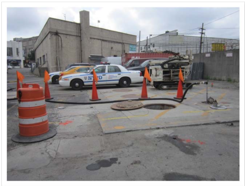
1. 46-81 Metropolitan Ave., Maspeth, NY – USTs Location
