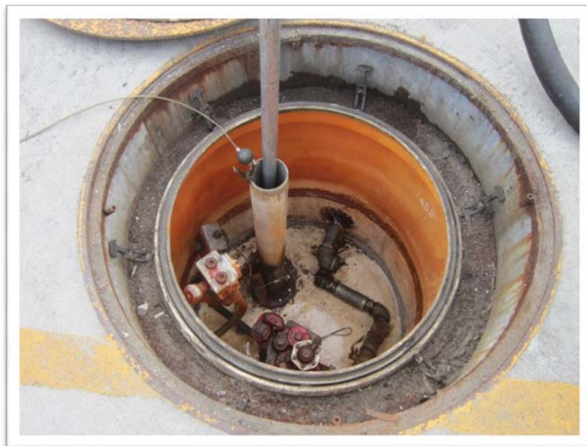
8. 4,000-gallon Gasoline UST After Cleaning Activity
