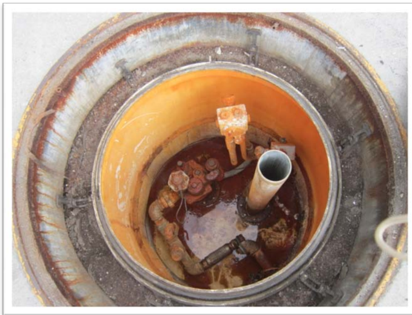
6. 4,000-gallon Gasoline UST Prior Cleaning Activity
