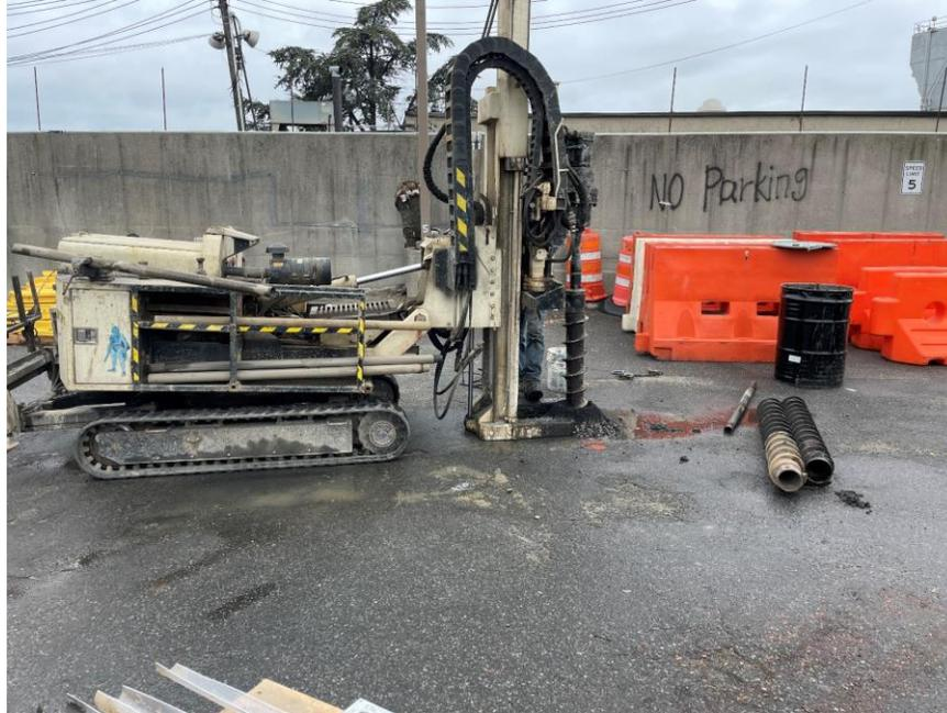
**Photo 1:** Lakewood using an auger to expand a borehole in preparation for monitoring well installation (facing east)
