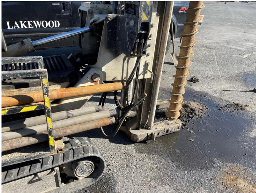
**Photo 2:** Lakewood using an auger to expand a borehole in preparation for monitoring well installation at soil boring SB17 (facing northwest)
