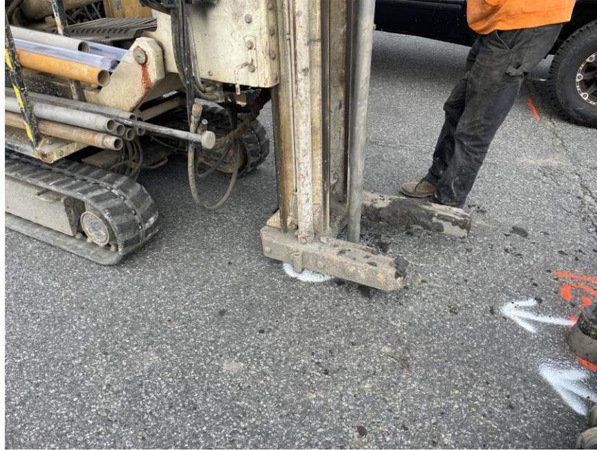
**Photo 1:** Lakewood advancing soil boring SB21 in the northwestern part of the site (facing northwest)
