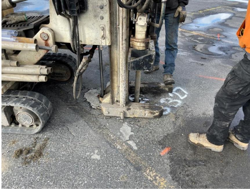
**Photo 1:** Lakewood advancing soil boring SB27 in the eastern part of the site (facing northwest)
