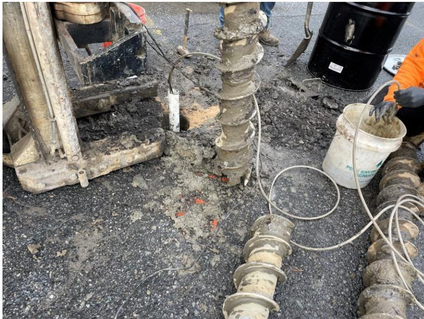
**Photo 2:** Lakewood developing monitoring well MW05 in the northwestern part of the site (facing northwest)
