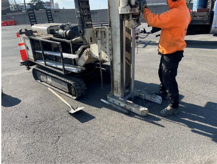
**Photo 1:** Lakewood advancing soil boring SB31 in the northern part of the site (facing southwest)
