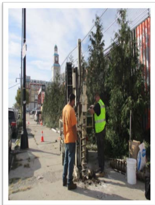
3. Monitoring Well Installation by Utilizing Geoprobe (6610DT)
