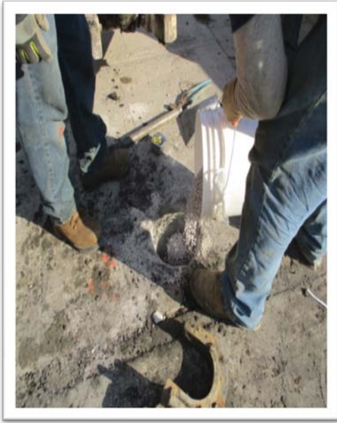
5. Placing the Bentonite Seal
