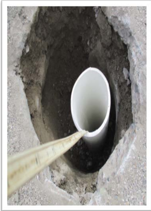
9. GW Level Measurement by Utilizing Water Level Meter
