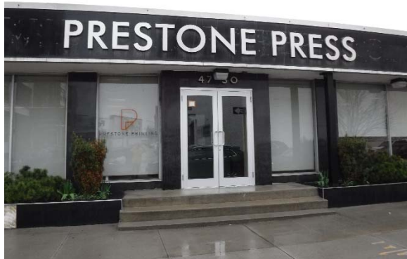
Photograph No. 1: Front view of the Subject Property located at 4750 30 th Street, Long Island City, NY
