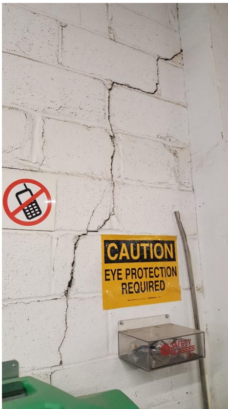
Photograph No. 5: View of northern exterior wall conditions
