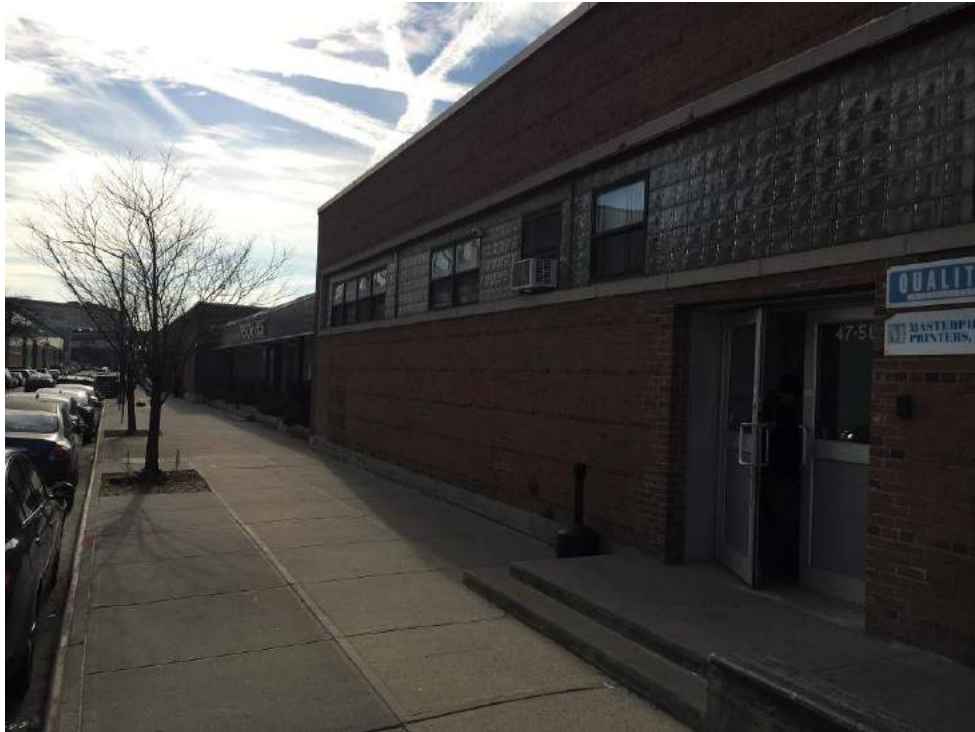
Photo 1: Front of building, facing southwest
