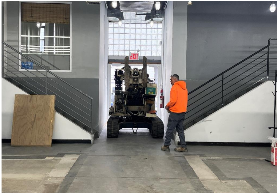
Photo 2: Geoprobe 7720DT entering the northern portion of the site building from an external door to 30 th Street.
