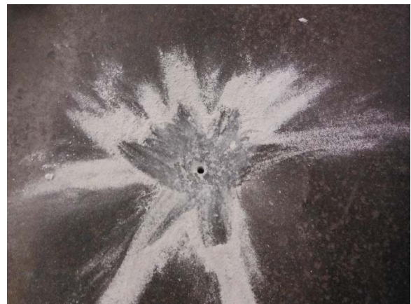
Photograph Nos. 4 & 5: The sub-slab vapor point was installed through the concrete slab of the main floor utilizing an electric-powered rotary hammer drill. Tubing was installed through the newly installed vapor point, and the point where the tubing entered the concrete slab was sealed with hydrated bentonite.
