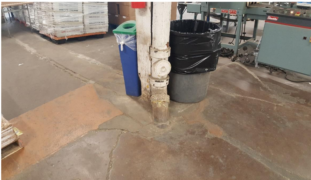
Photograph No. 4: Representative view of interior drilling locations
