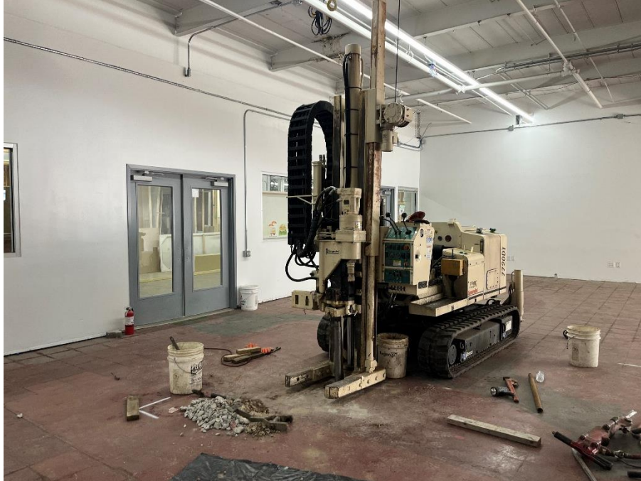
Photo 1: Geoprobe 7720DT at SB14
