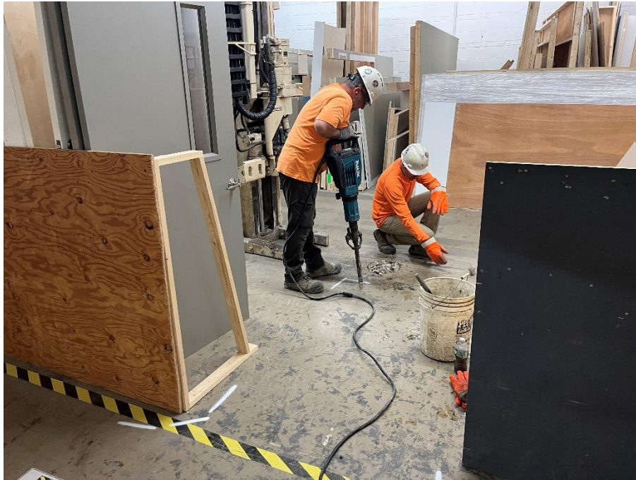
Photo 1: Breaking the concrete slab at boring SB04.
