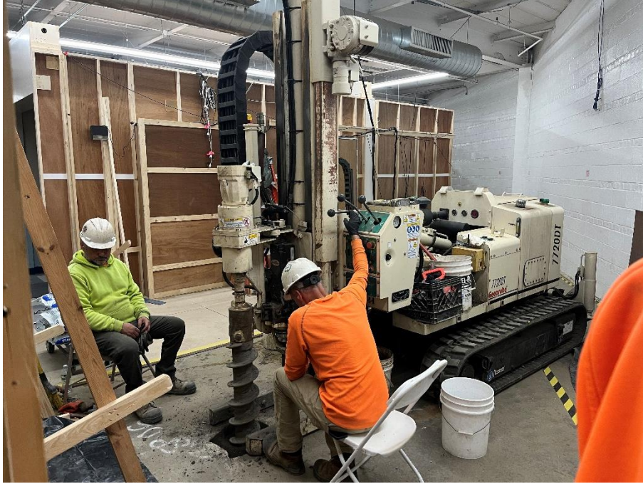
Photo 1: Geoprobe 7720DT augering monitoring well MW-6.
