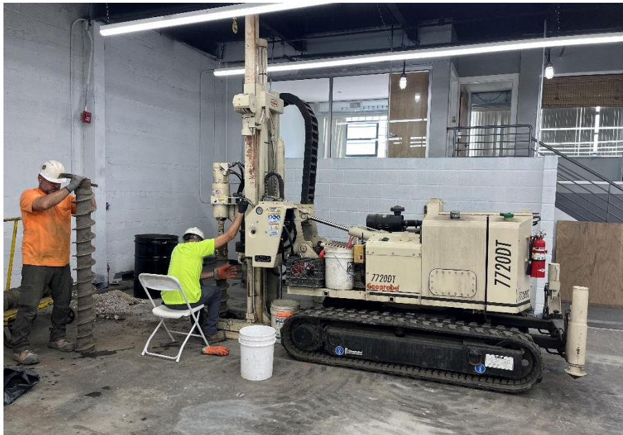
Photo 2: Geoprobe 7720DT augering permanent monitoring well MW-2.
