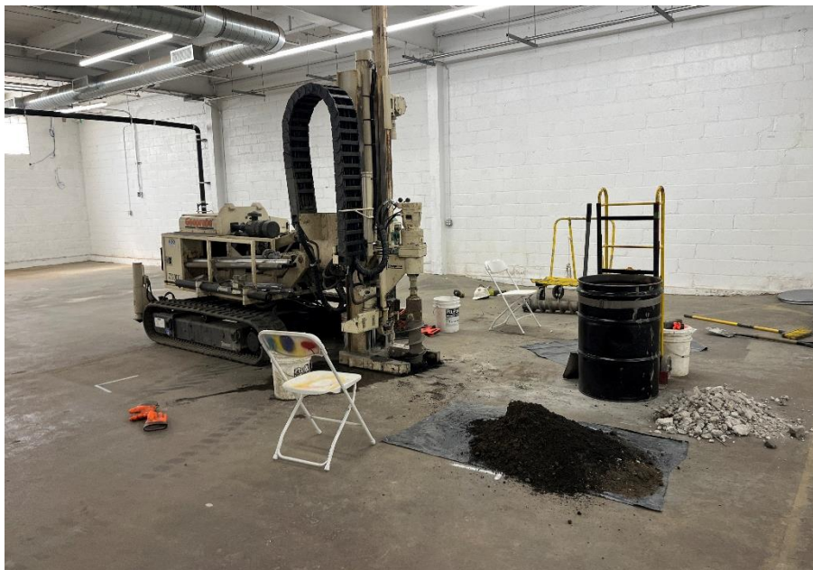
Photo 2: Geoprobe 7720DT augering monitoring well MW-1.
