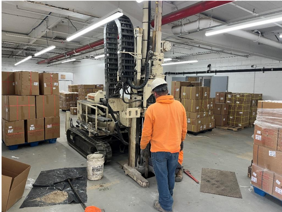
Photo 1: Geoprobe 7720DT advancing soil boring SB12.
