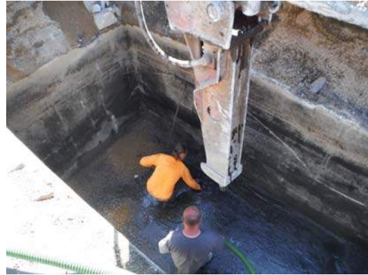
Photograph Nos. 10 & 11 - As discussed with the NYSDEC, two (2) bottom samples were collected through the concrete floor of the vault in order to determine the environmental condition of underlying soils.
