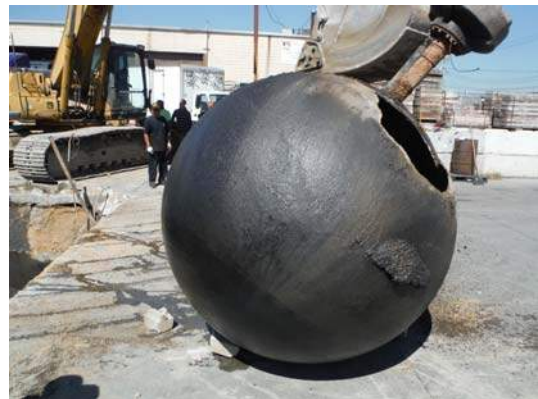
Photograph Nos. 5 & 6- Inspection of the 4,000-gallon single-wall fiberglass UST noted the absence of any holes or cracks that did not appear to be sustained during the removal efforts.
