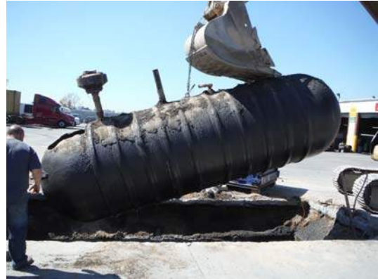
Photograph No. 4 – Upon completion of the removal of all liquids from within the UST, the UST subsequently removed from the ground.
