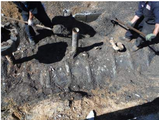
Photograph No. 3 – While uncovering the UST, stained pea-gravel exhibiting diesel fuel odors and elevated PID readings were observed surrounding the former fill piping. The NYSDEC was notified and Spill No. 13-06438 was assigned to the property.
