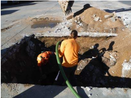
Photograph No. 2 – Prior to the removal of the 4,000-gallon Diesel UST, approximately 350 gallons of residual diesel and sludge was removed from within UST via a pump truck for proper disposal.
