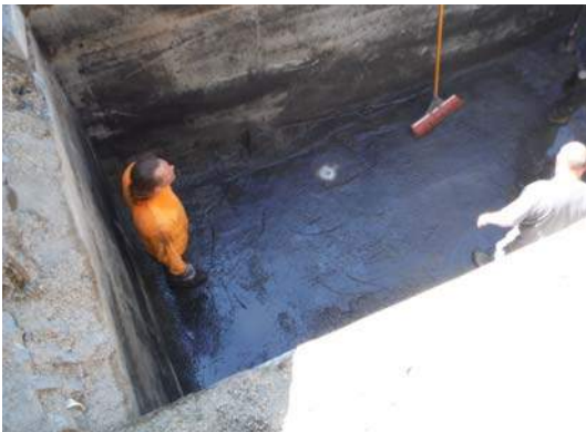
Photograph Nos. 8 & 9 - Both the pea-gravel and trapped water were removed from within the vault for off-site disposal.
