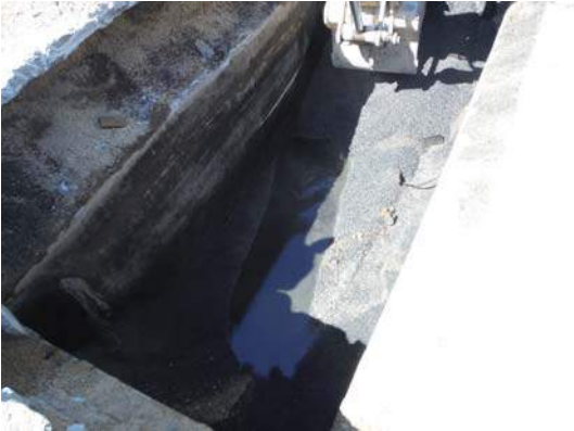
Photograph Nos. 8 & 9 - Both the pea-gravel and trapped water were removed from within the vault for off-site disposal.
