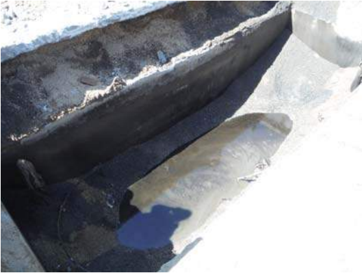
Photograph No. 7 – The UST was contained within a solid concrete vault extending to twelve (12) feet below grade surface (bgs). Pea-gravel and trapped water contained within the vault was noted to contain diesel fuel odors, staining and exhibited elevated Photoionization Detector (PID) responses.
