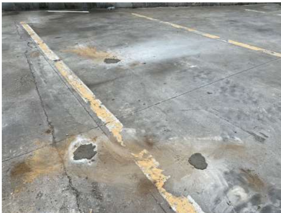
Photograph 8: View of the final site restoration using Portland cement at soil boring SB04 (facing east)
