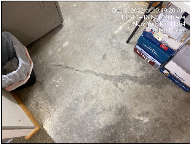
Sealed floor cracks in the southern portion of the building's basement near the boiler room.
