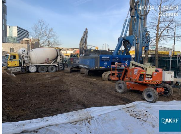
Photograph 1 - Grouting soldier piles in Grid WC-6, view facing west.
