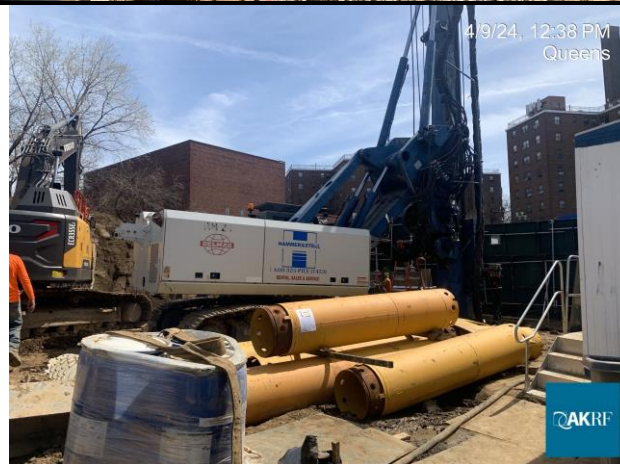
Photograph 3- Drill assembly in Grid WC-4, view facing southeast.
