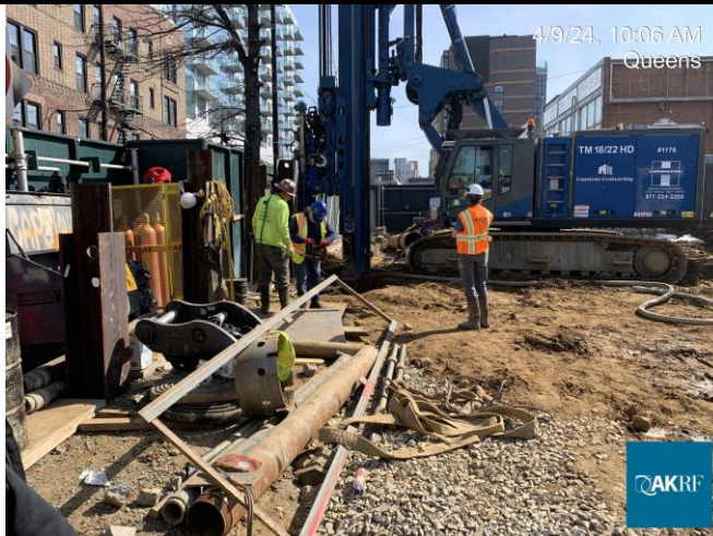
Photograph 2- Drilling soldier piles in Grid WC-6, view facing east.
