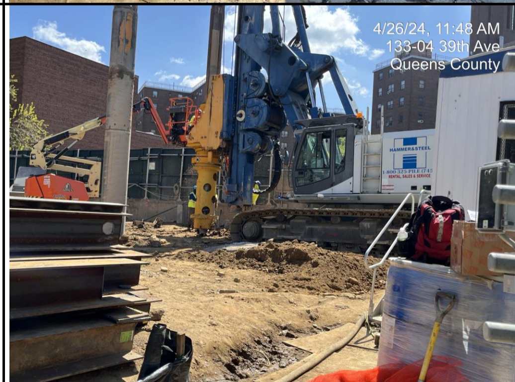
Photograph 3 - Drilling piles in Grid WC-7, view facing southeast.
