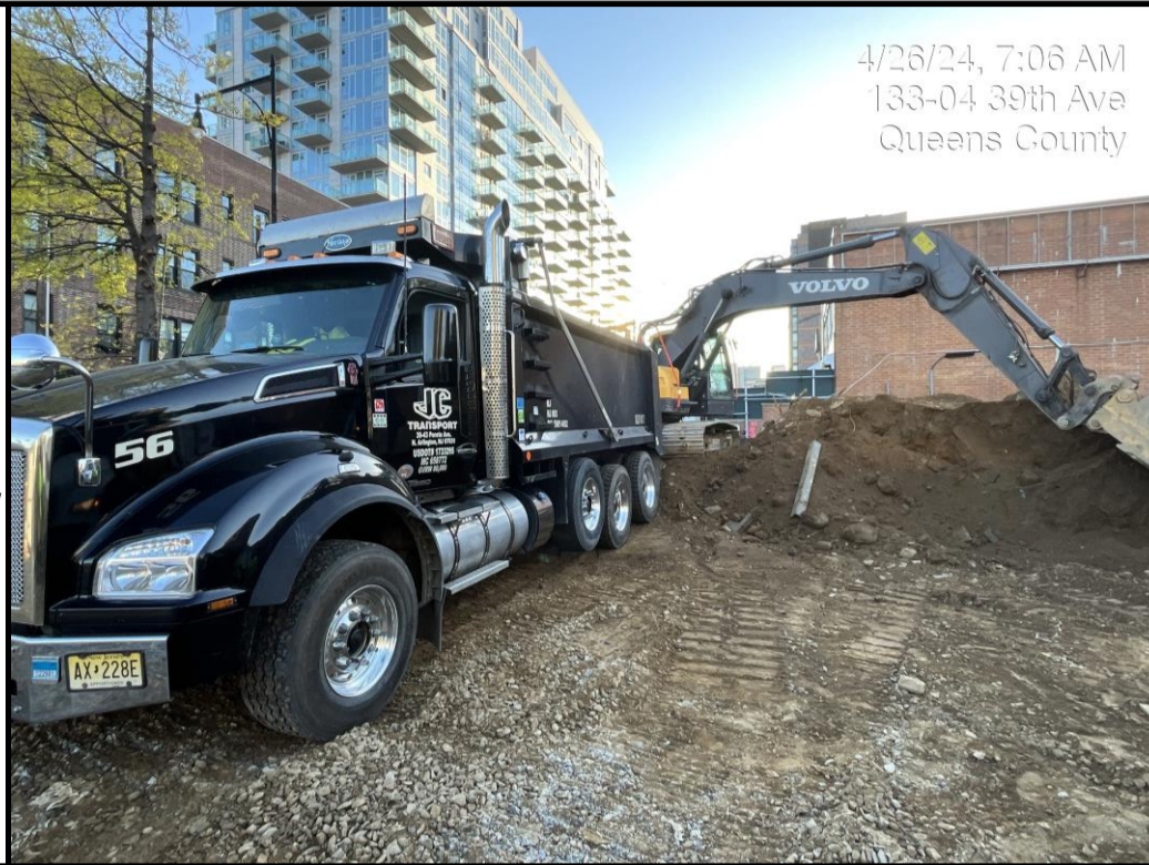
Photograph 1 - Loading truck with non-hazardous soil for off site disposal from Grid WC-3. View facing east.
