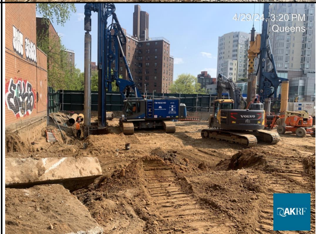
Photograph 3 - Drilling piles in Grids WC-3 and 4, view facing south.
