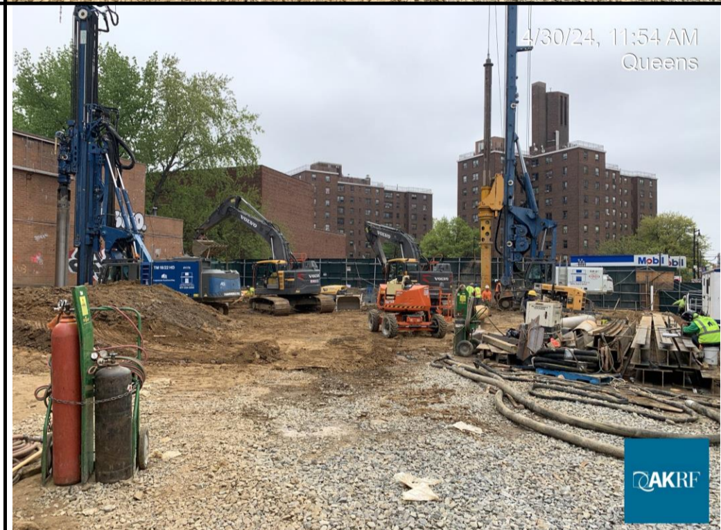
Photograph 2 - Site overview. View facing southeast.
