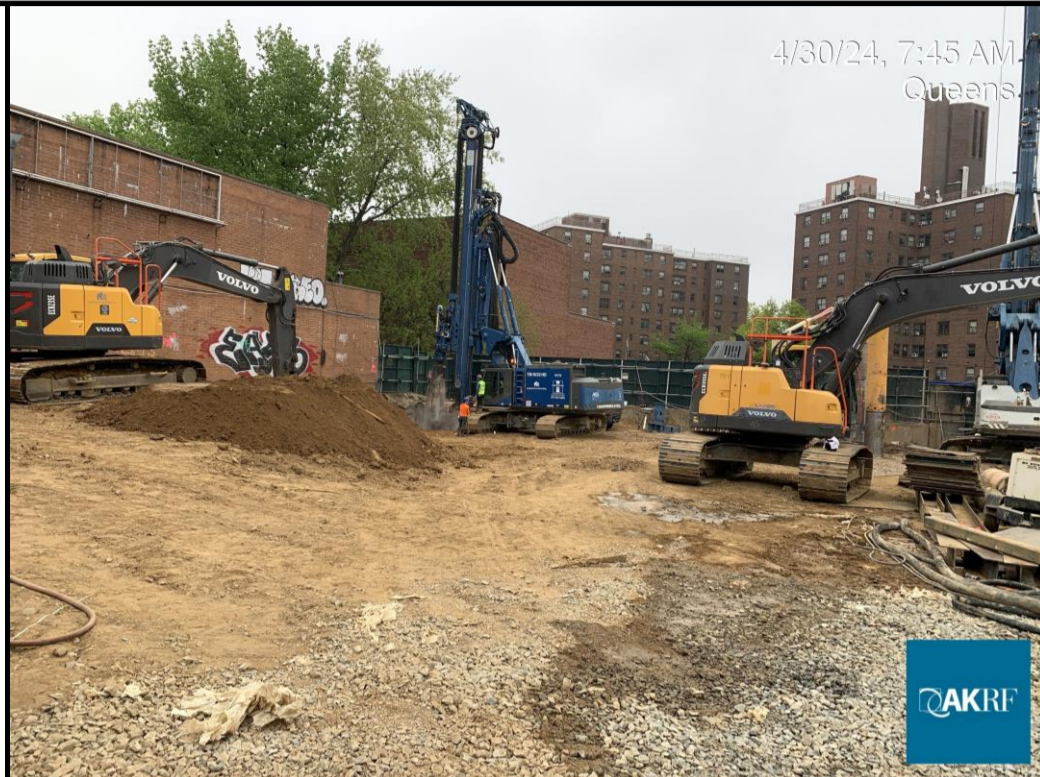
Photograph 1 - Drilling piles in WC-3. View facing southeast.
