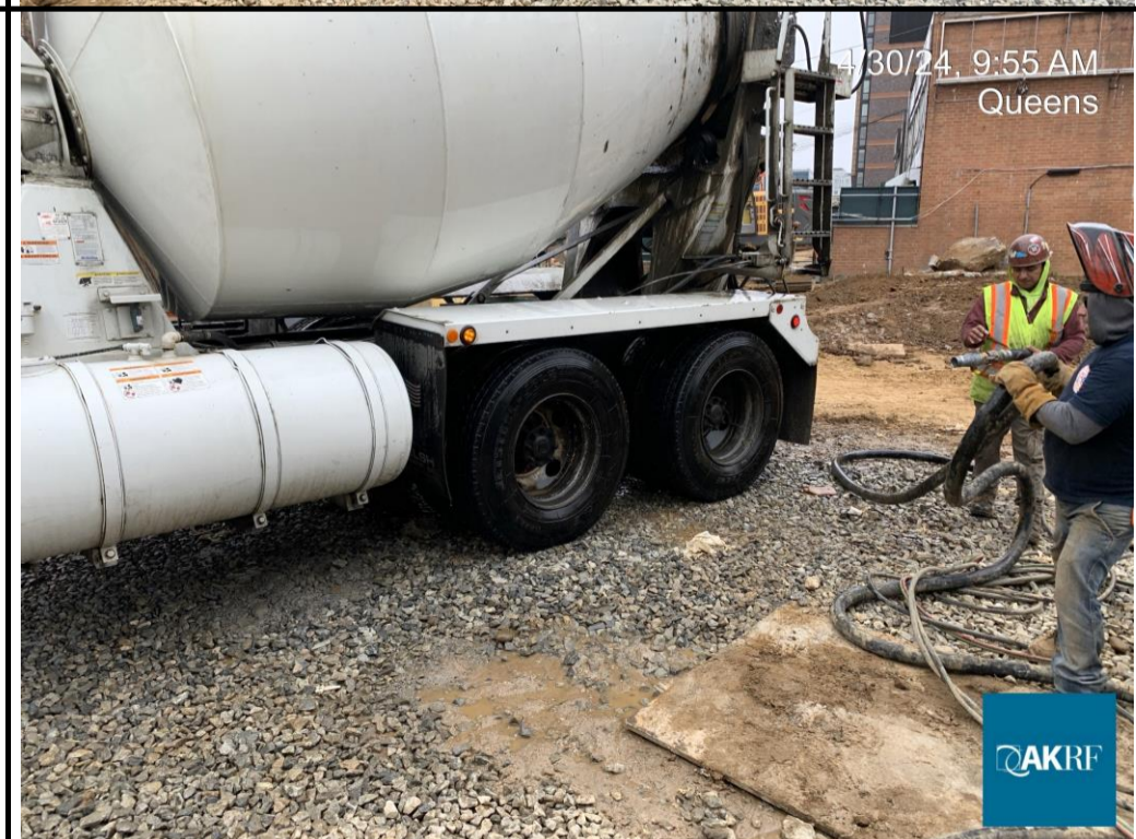
Photograph 3 - Washing truck tires before leaving the site, view facing east.
