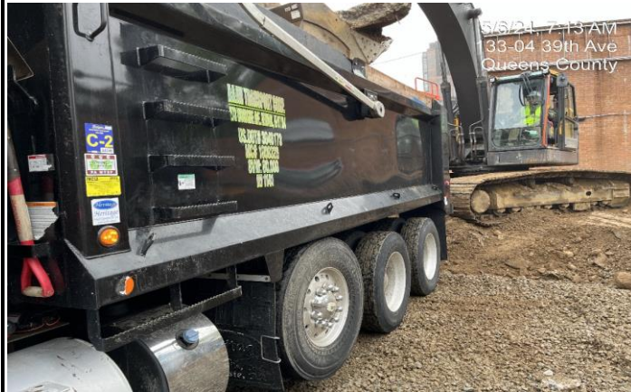
Photograph 1 - Non-hazardous soil being loaded for disposal.
