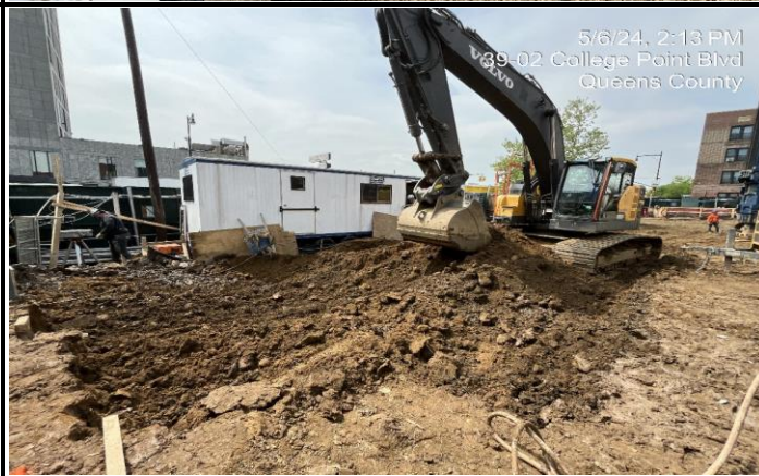
Photograph 2 - Excavating soil in WC- 4.
