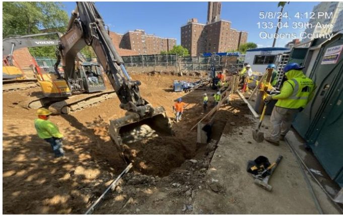
Photograph 2 - Lagging installation in Grid WC-4.
