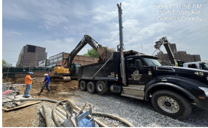
Photograph 1 - Non-hazardous soil being loaded on to trucks for disposal.
