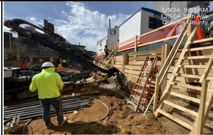
Photograph 2 - Drilling tiebacks for SOE in Grid WC-4.
