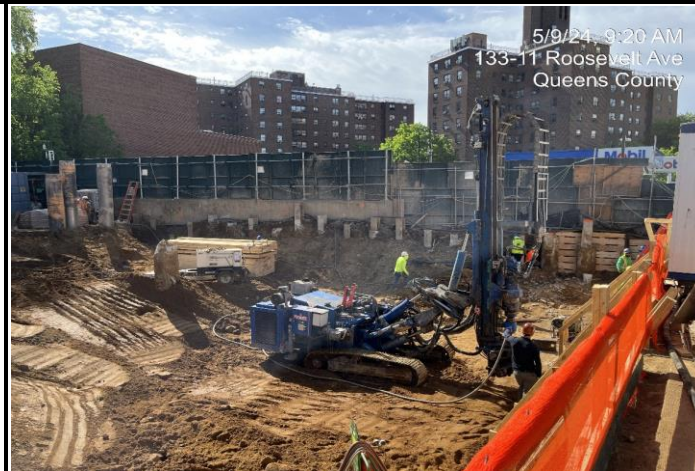
Photograph 3 - Installing SOE in Grid WC-4.
