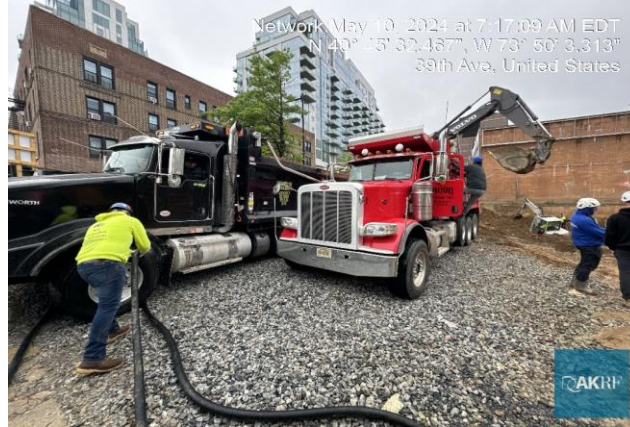
Photograph 1 - Non-hazardous soil being loaded on to trucks for disposal.
