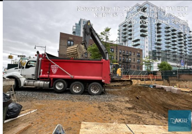
Photograph 2 - Non-hazardous soil being loaded on to trucks for disposal
