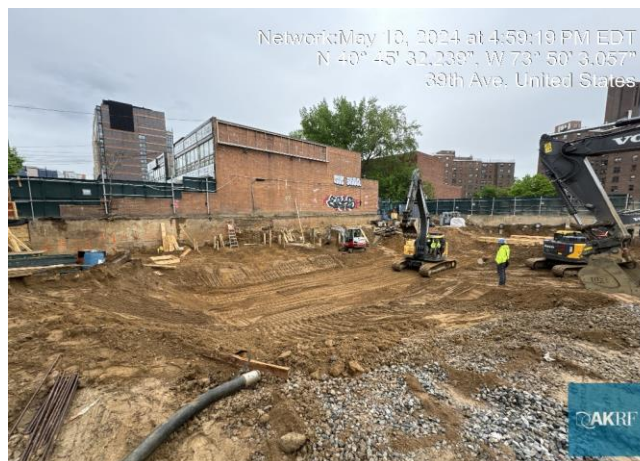
Photograph 3 - Excavating/grading in Grid WC-3.
