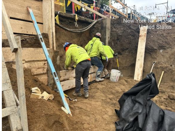
Photograph 1 - Lagging installation in Grid WC-4.
