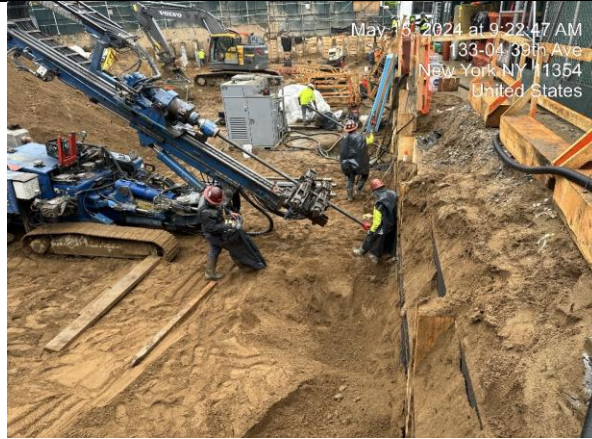
Photograph 2 - Drilling for tiebacks in Grid WC-2.
