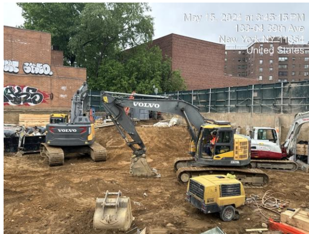
Photograph 3 - Grading in Grid WC-8.
