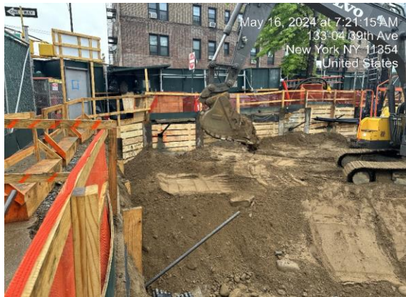
Photograph 1 - Relocating and constructing the truck ramp in the northern portion of the Site.
