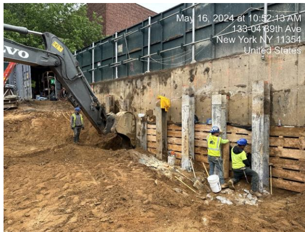
Photograph 3 - Excavation for SOE in WC-8.
