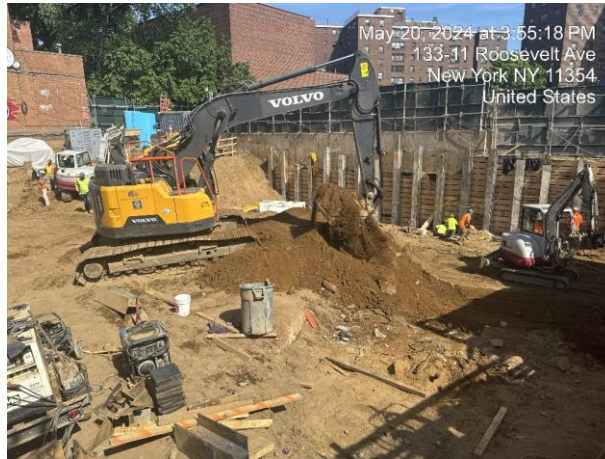
Photograph 3 - Excavation in Grid WC 7.
