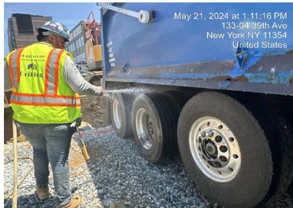
Photograph 3 - Truck tires being washed upon exiting Site in Grid WC-2. Wash water was collected in the collection pit.
