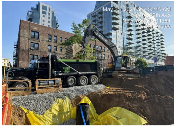
Photograph 2 - Non-hazardous soil being loaded on to trucks for export to Bayshore.
