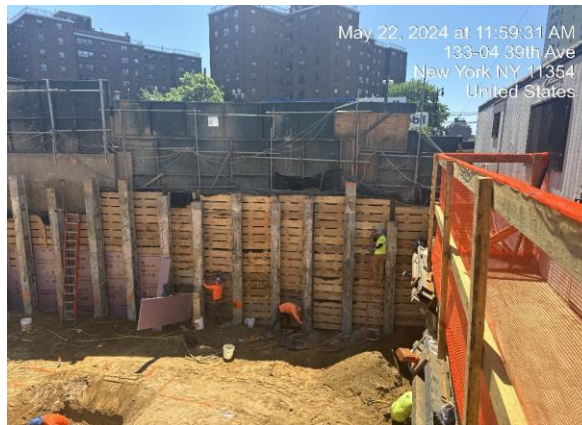
Photograph 3 - Lagging installation for SOE in Grid WC-4.
