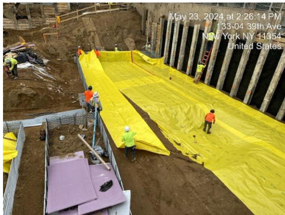
Photograph 2 - Installing 20-mil Stego Wrap vapor barrier in the southwestern portion of Site.
