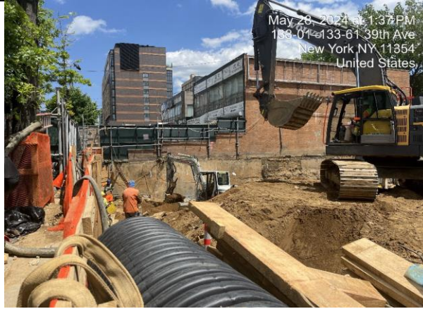
Photograph 1 - SOE related excavation in Grids WC-1 and WC-5.
