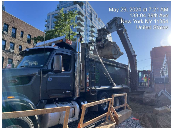
Photograph 3 - Loading soil on to trucks for off-site disposal.
