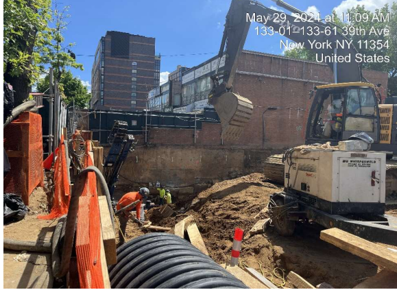
Photograph 1 - SOE related excavation in WC-1/5.
