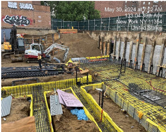
Photograph 2 - Contractor installed rebar in the southwestern portion of the Site as part of the foundation construction.
