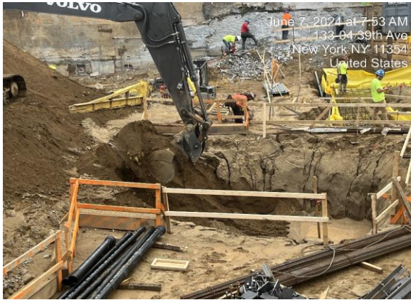
Photograph 2 - Excavation and grading in Grid WC-01 for installation of elevator.
