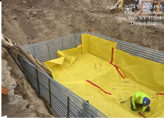
Photograph 1 - Vapor Barrier installation in Grid WC-01, facing north.
