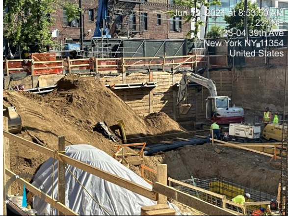
Photograph 1 - Excavation and grading in WC-5 for lagging installation, view facing northeast. Soil stockpile remains covered with poly sheeting.
