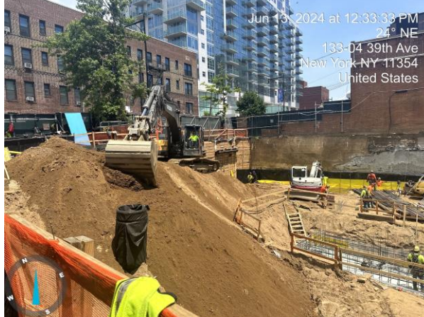
Photograph 2 - Excavation and grading in WC-1/5/6, view facing northeast.
