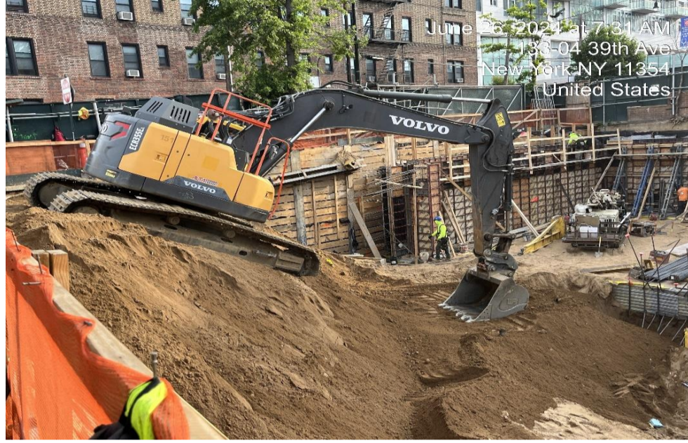
Photograph 1 - Grading in WC-1 for site work. View facing northeast.
