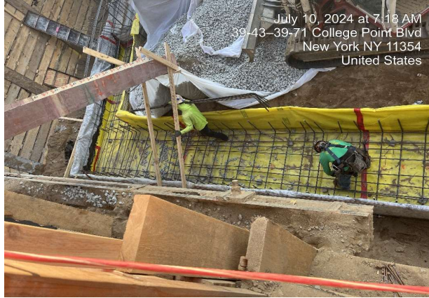
Photograph 1 - Installation of vapor barrier in Grids WC-2/6, facing northwest.
