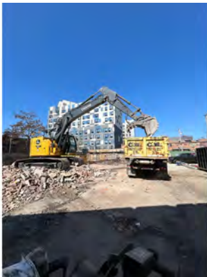
Construction debris removal (April 24)
