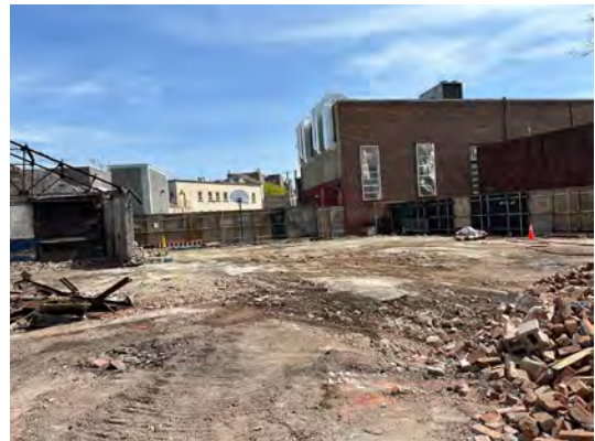
Site post-demolition (April 24)
